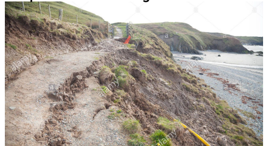
Footpath erosion leading to mass movement
